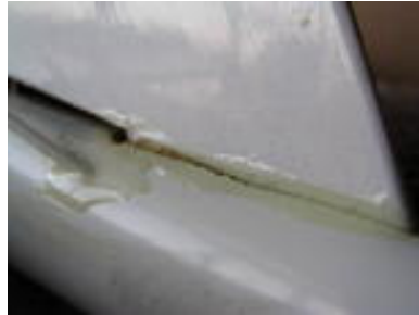
Note location of cable drilling
